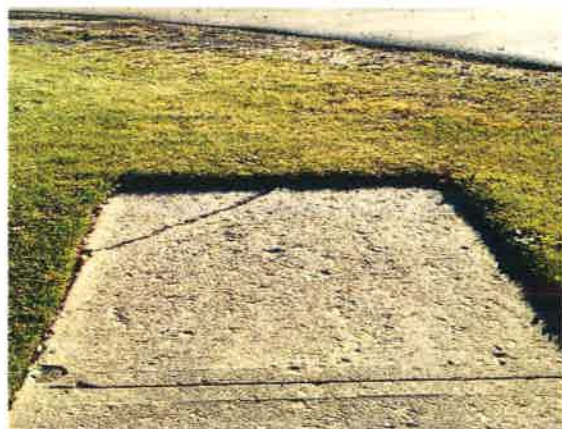
Corner Break: Segment/Asset_Id 332613N
