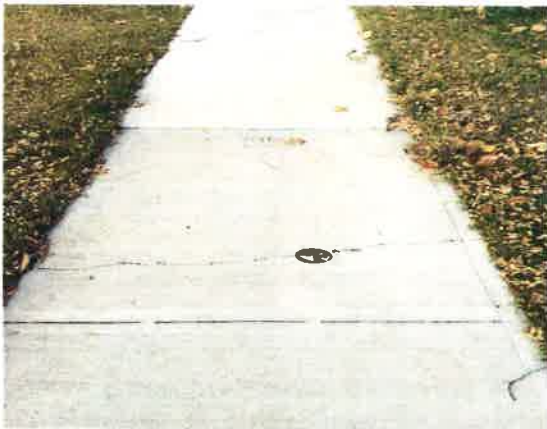
Linear Cracking: Segment/Asset_Id 165619N
