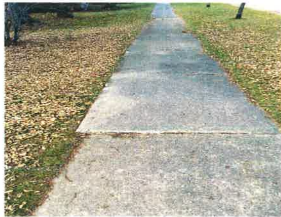
Faulting: Segment/Asset_Id 61643S
