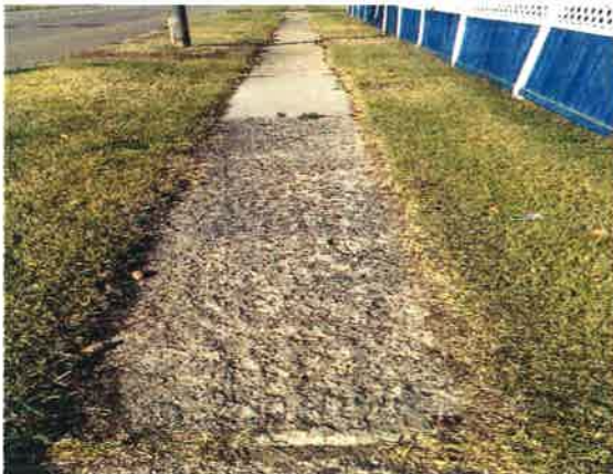
Scaling: Segment/Asset_Id 123243N
